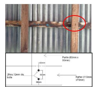
Fig.12 Purlin to rafter connection detailings.
